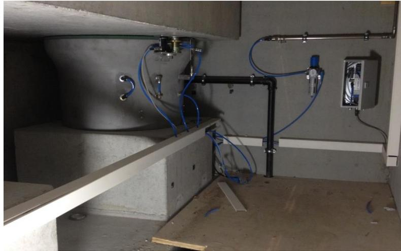
**Fig. 4: Membrane air springs BiAir® 5-ED/HE-Max under the foundation block**
