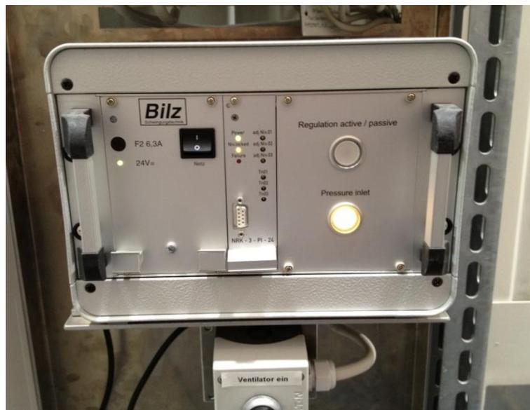
**Fig. 3: Level monitoring system installed outside the chamber**
